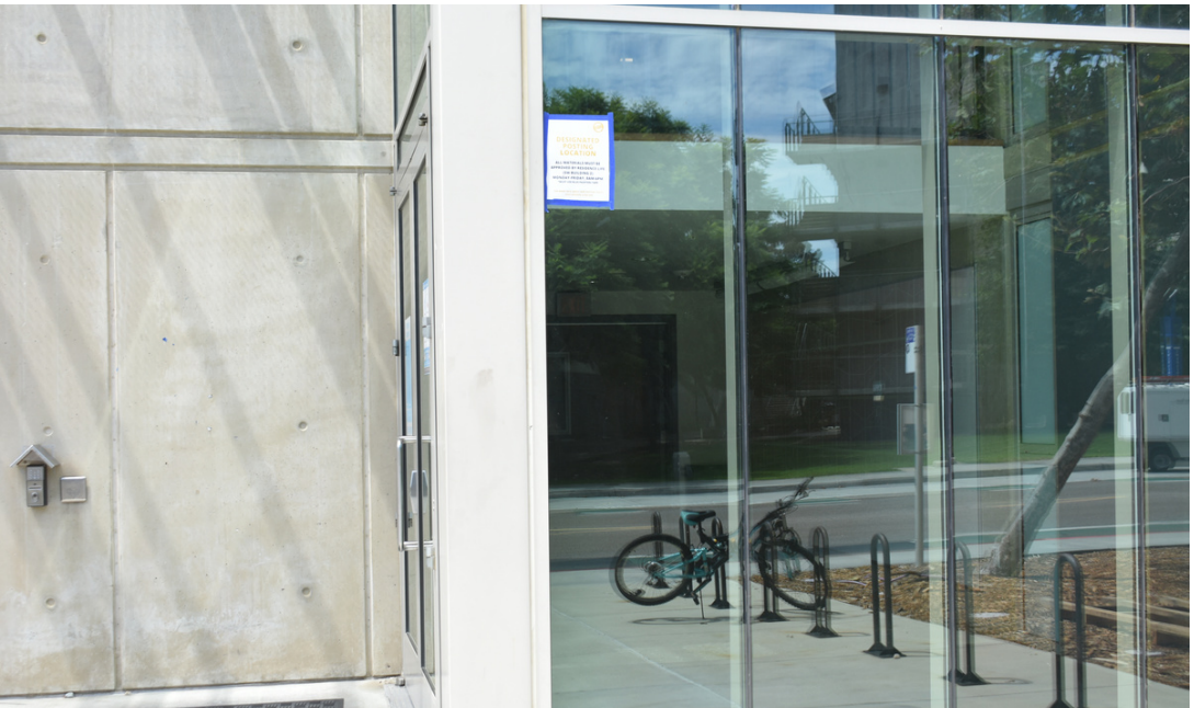
Second floor entrance
