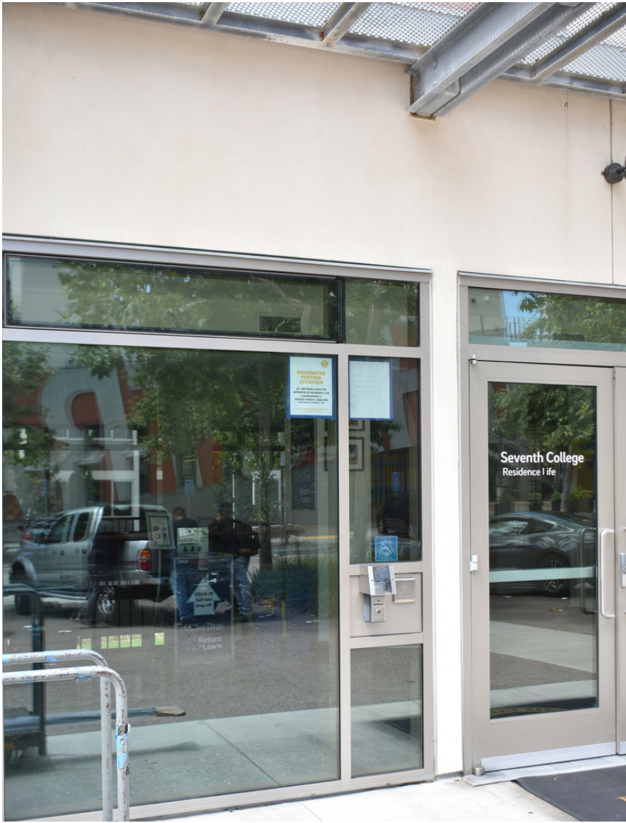
Second floor entrance
